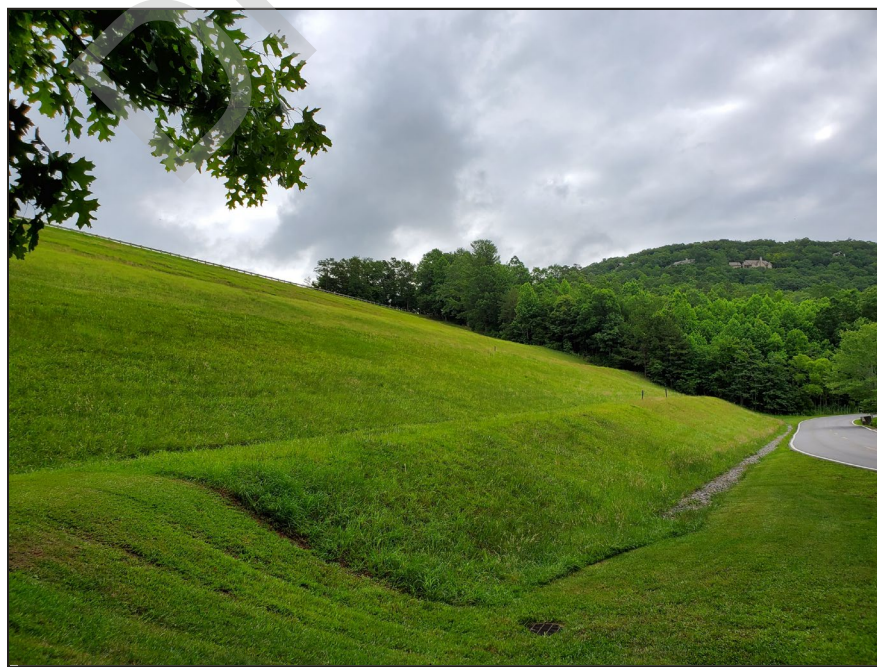
Photograph 2: Downstream Face, June 2020 – overview of downstream face in good condition
