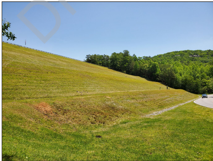
Photograph 2: Downstream Face, May 2020 – overview of downstream face in good condition
