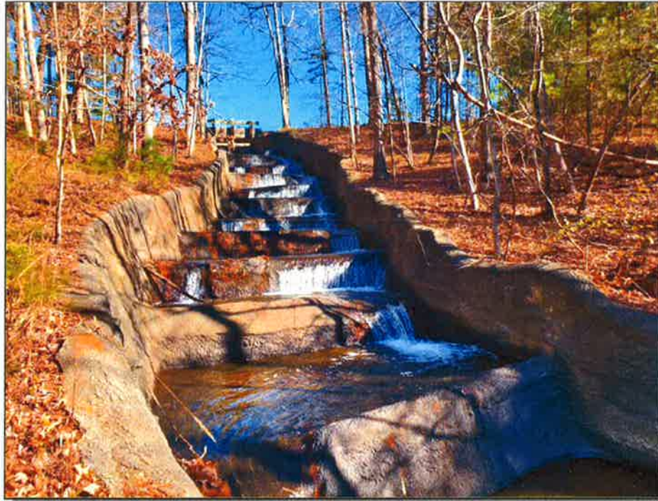
Photograph 3: Spillway, Nov. 2020 – general view of stepped spillway with moderate flow, and tree limbs and debris noted during inspection.
