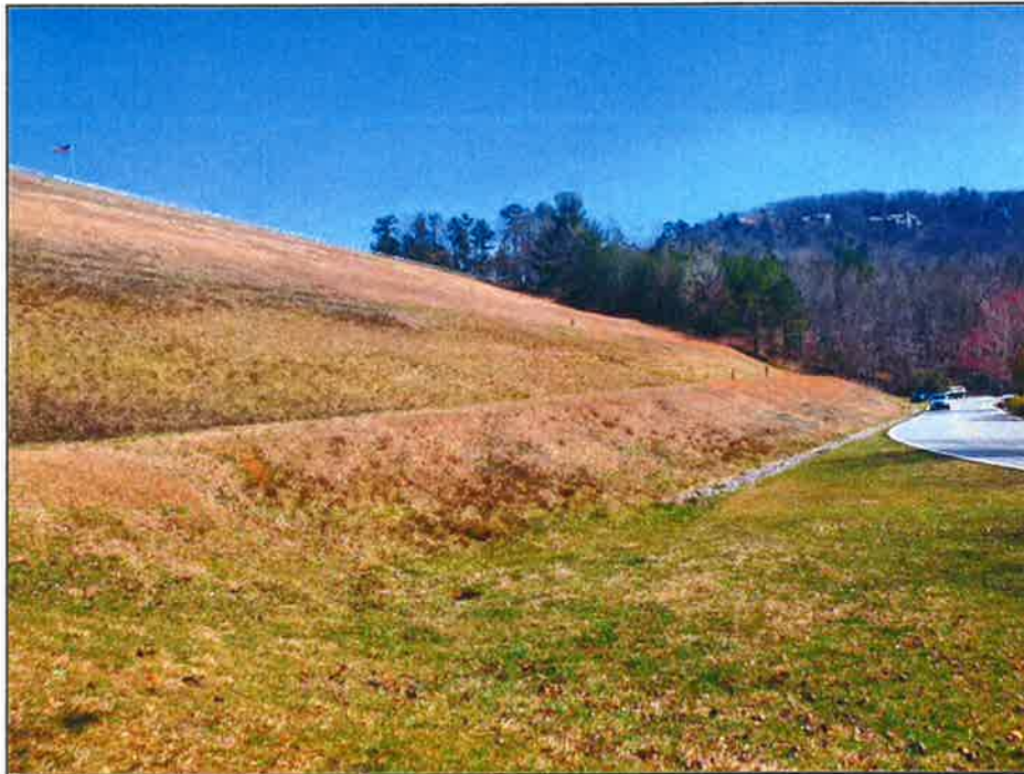
Photograph 2: Downstream Face, Mar. 2021 – overview of downstream face in good condition
