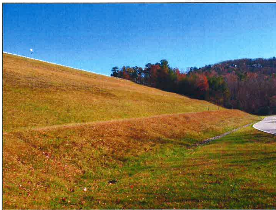
Photograph 2: Downstream Face, Nov. 2020 – overview of downstream face in good condition
