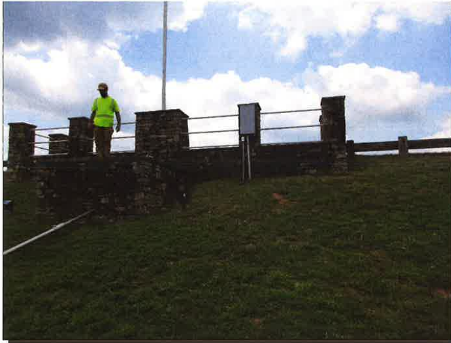
Photograph 1: View of the low-level valve box
