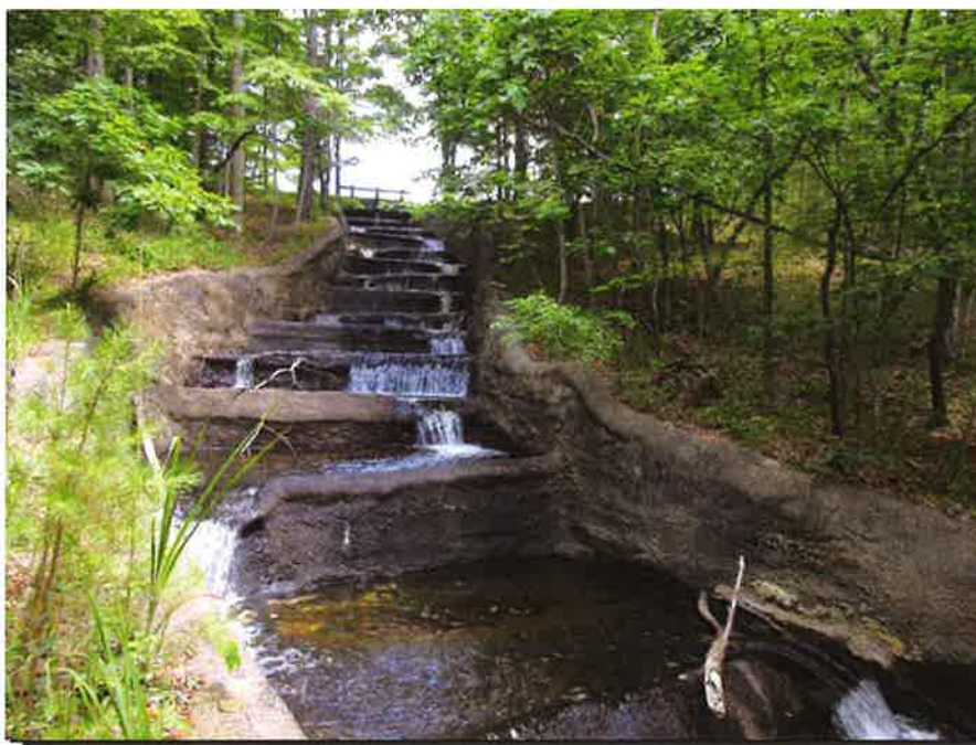
Photograph 4: Spillway, 2016 – general view with moderate flow during observation
