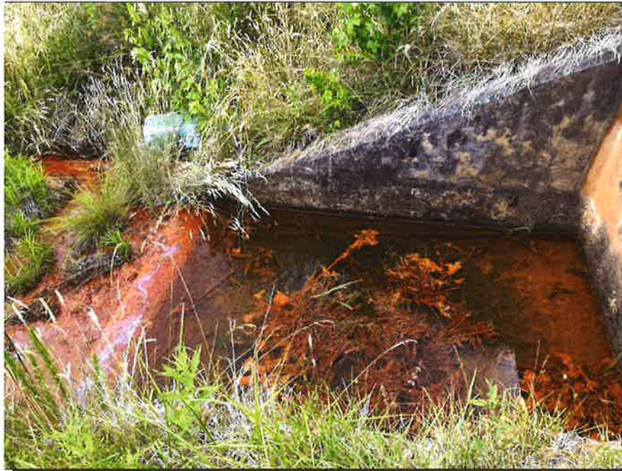
Photograph 3: Tail Water Creek, 2016 – Low-level drain outlet.
