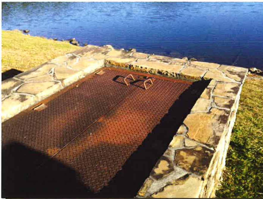
Photograph 2: View of the low-level valve box.
