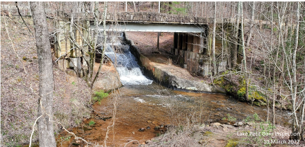
Photograph 30: Overflow Spillway discharge into Petit Creek
