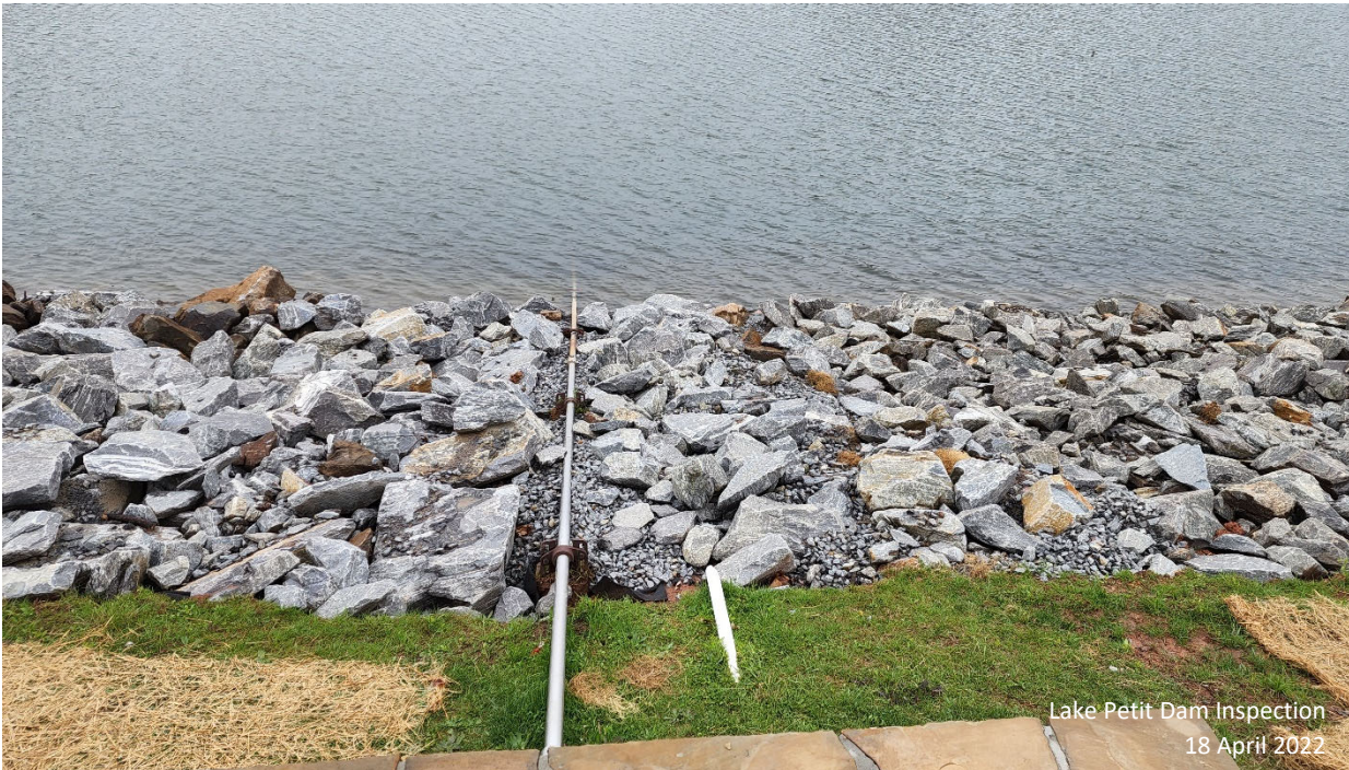
Photograph 5: Shoreline protection repairs completed (looking down alignment of gate stem)
