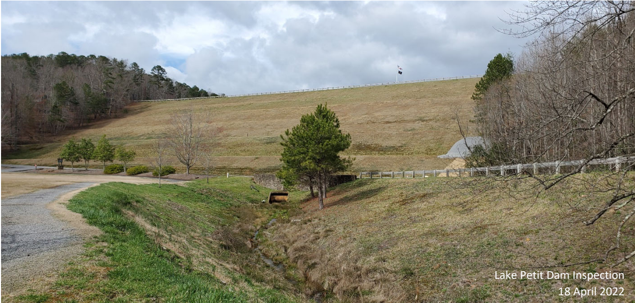
Photograph 31: Downstream slope and cleared channel below stilling basin discharge
