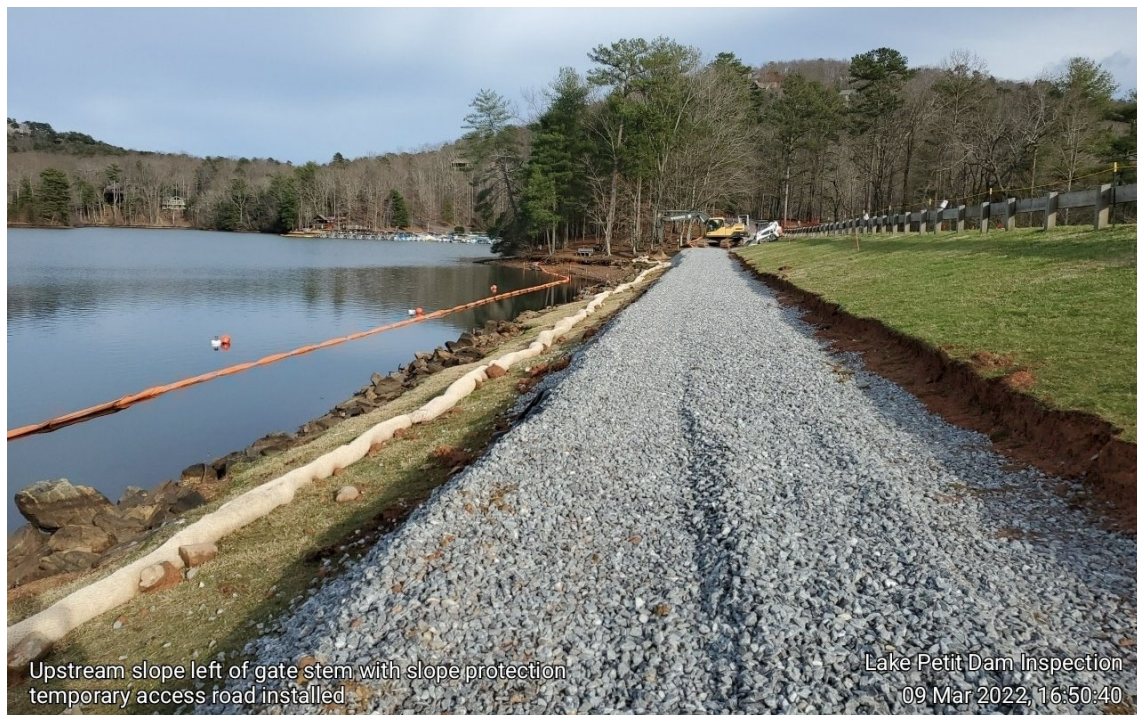
Photograph 2: Temporary access road for shoreline protection repairs
