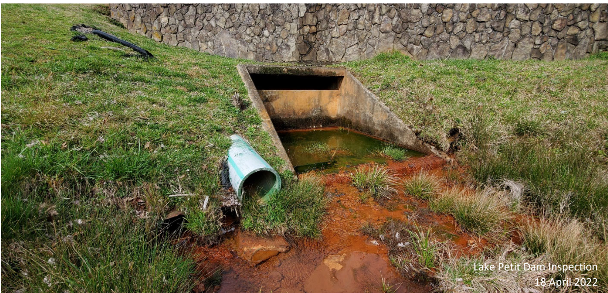
Photograph 32: Stilling basin discharge area
