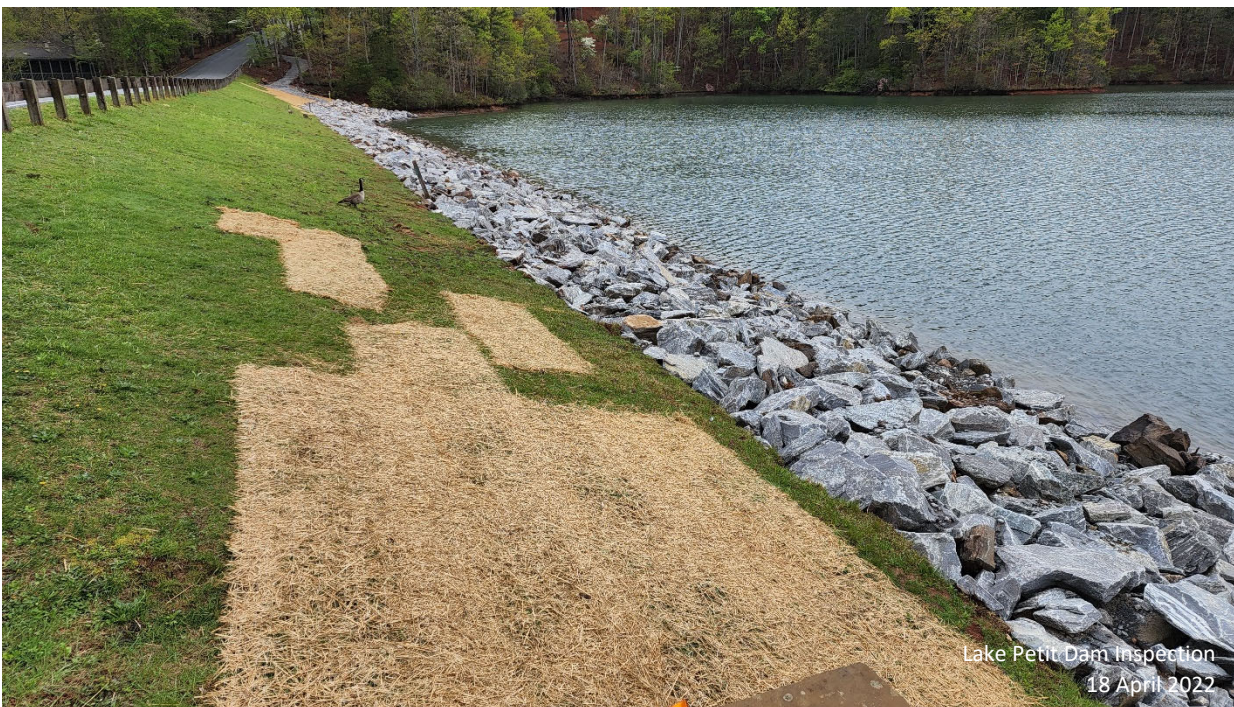
Photograph 6: Shoreline protection repairs completed (looking toward right abutment)
