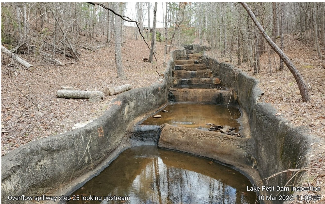
Photograph 27: Partially dewatered spillway looking upstream from Step 25
