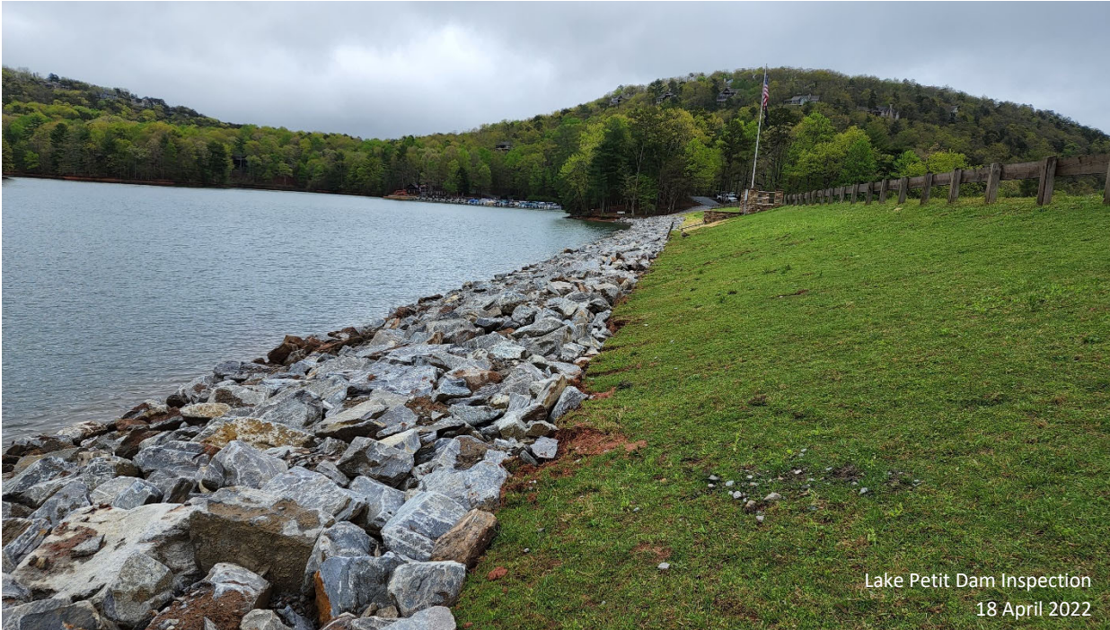
Photograph 7: Shoreline protection repairs completed (looking toward left abutment)
