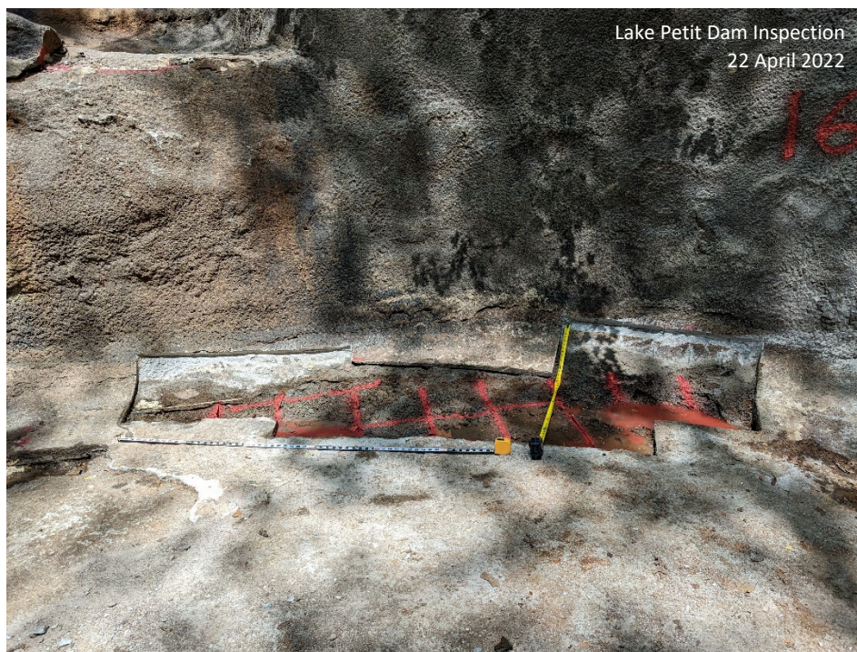
Photograph 36: Repair at Step 16 – removal of damaged gunite section
