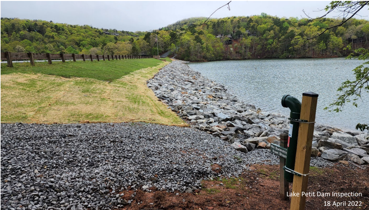
Photograph 3: Shoreline protection repairs completed (looking toward right abutment)
