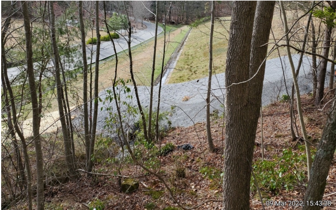
Photograph 15: Seepage area repair from left abutment
