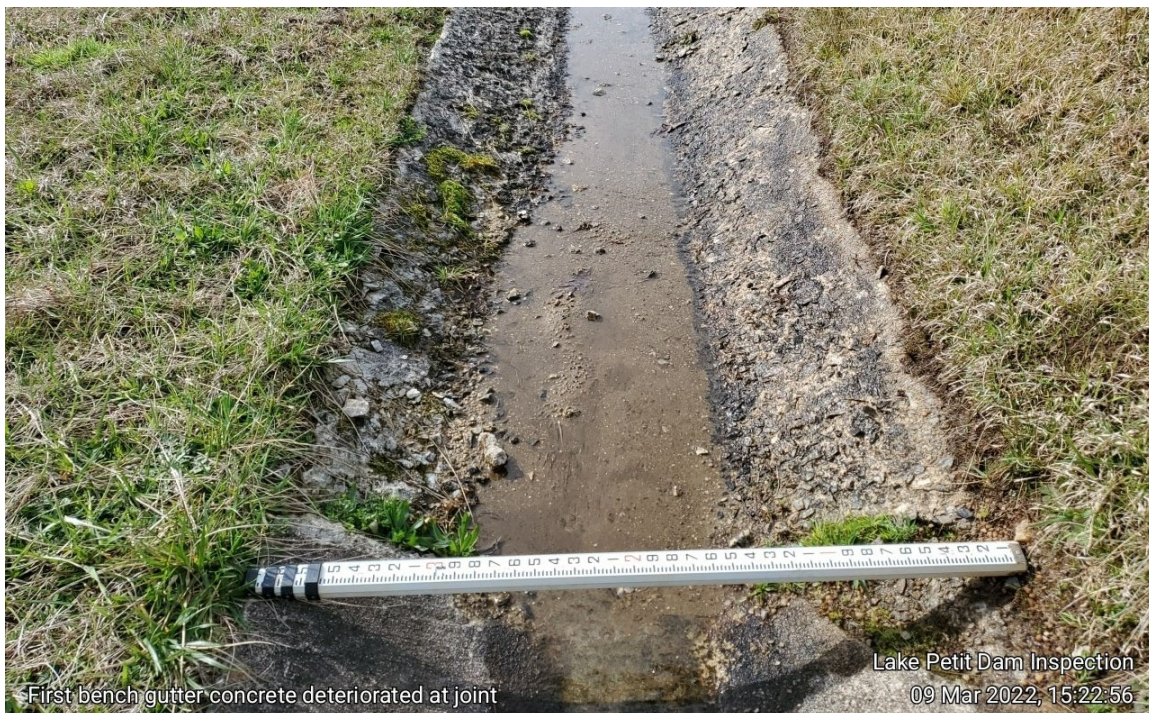
Photograph 18: Concrete drainage channel on Bench 1 (El. 1544)
