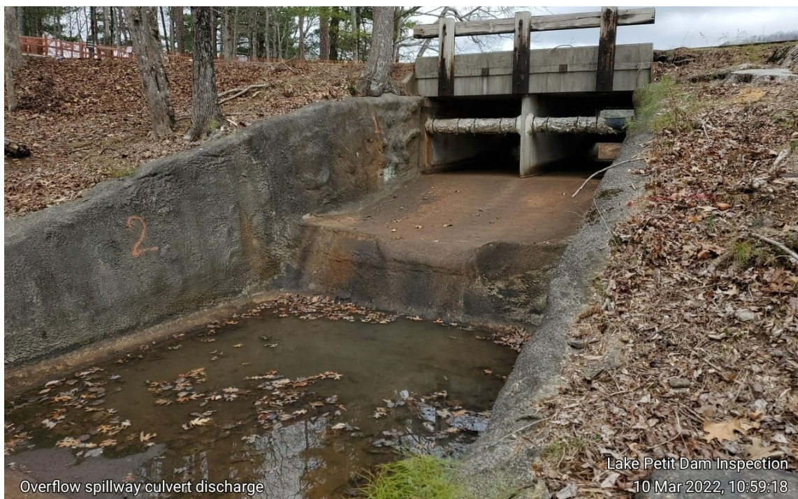
Photograph 26: Downstream side of box culvert
