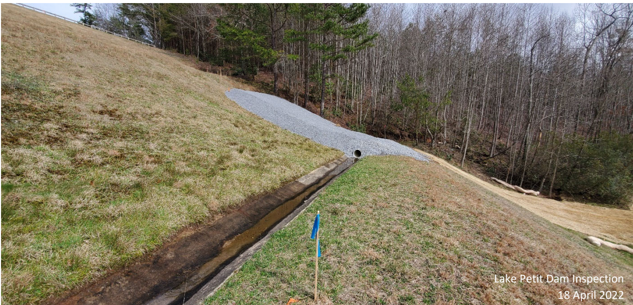
Photograph 16: Seepage Area Repair between Bench 1 (El. 1544) and Bench 2 (El. 1562)
