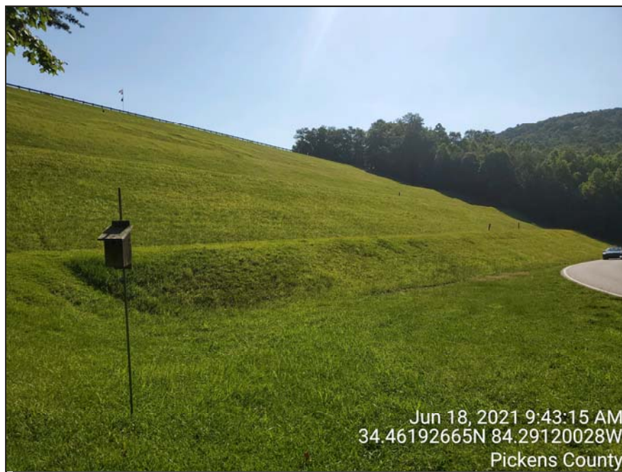
Photograph 2: Downstream Face, Jun. 2021 – overview of downstream face in good condition
