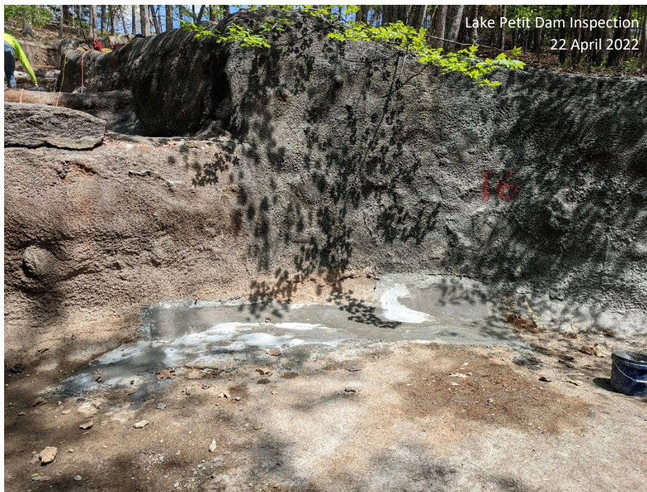
Photograph 38: Repair at Step 16 – repair complete
