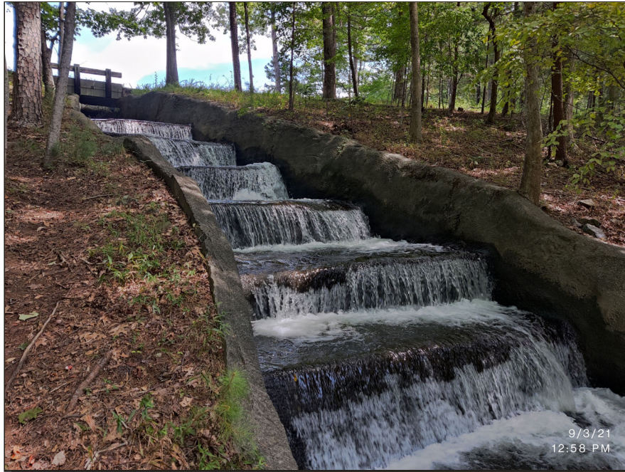
Photograph 3: Spillway, Sept. 2021 – general view of stepped spillway with moderate flow.
