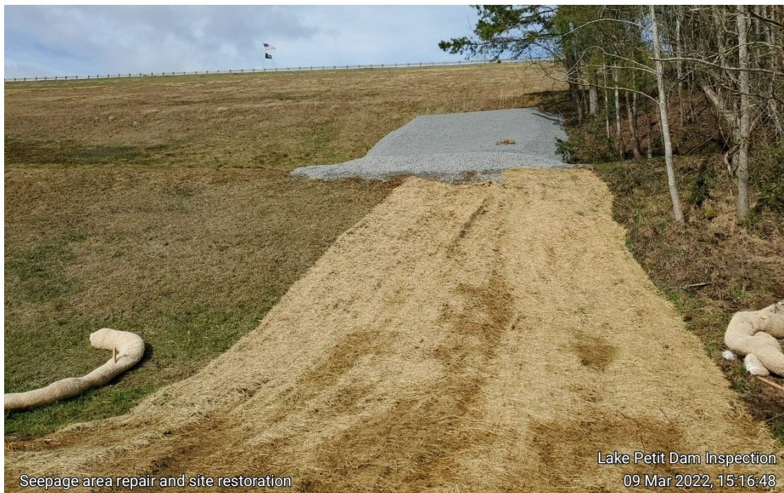
Photograph 14: Seepage area repair and site restoration
