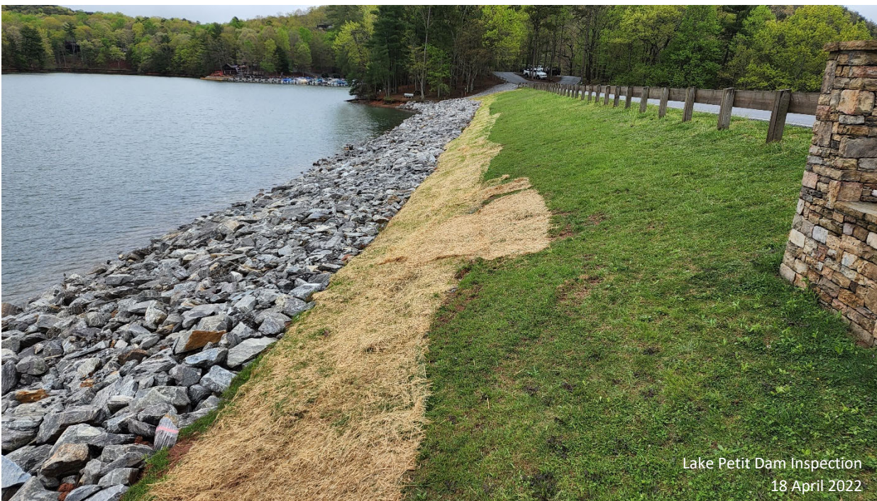
Photograph 4: Shoreline protection repairs completed (looking toward left abutment)
