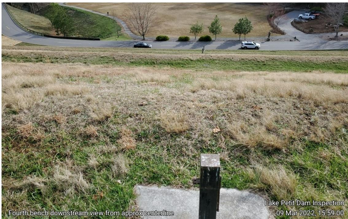
Photograph 21: Bench 4 (El. 1606) looking downstream from midpoint of alignment
