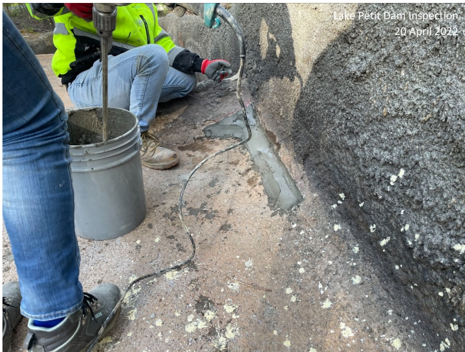
Photograph 35: Cracked area patched
