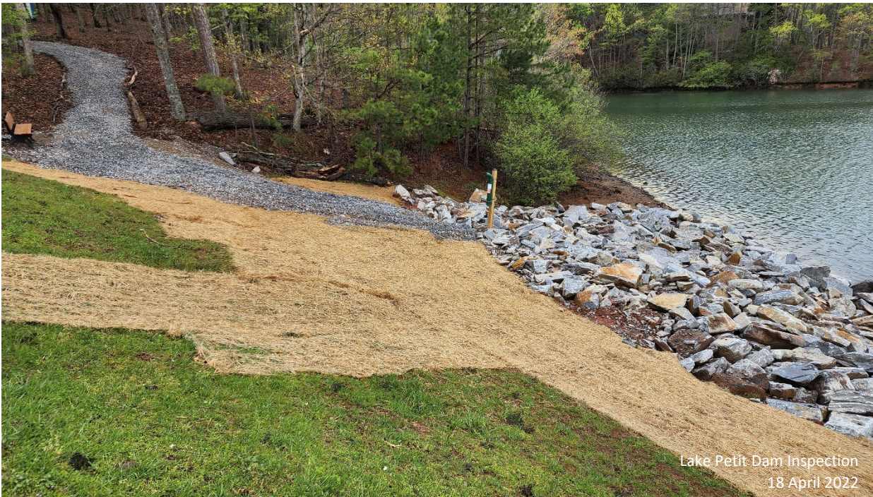
Photograph 8: Shoreline protection repairs and new pedestrian access on right abutment
