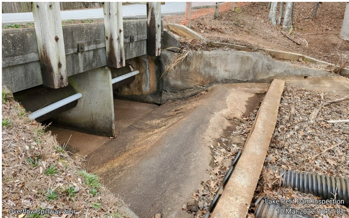
Photograph 25: Overflow spillway crest weir and box culvert
