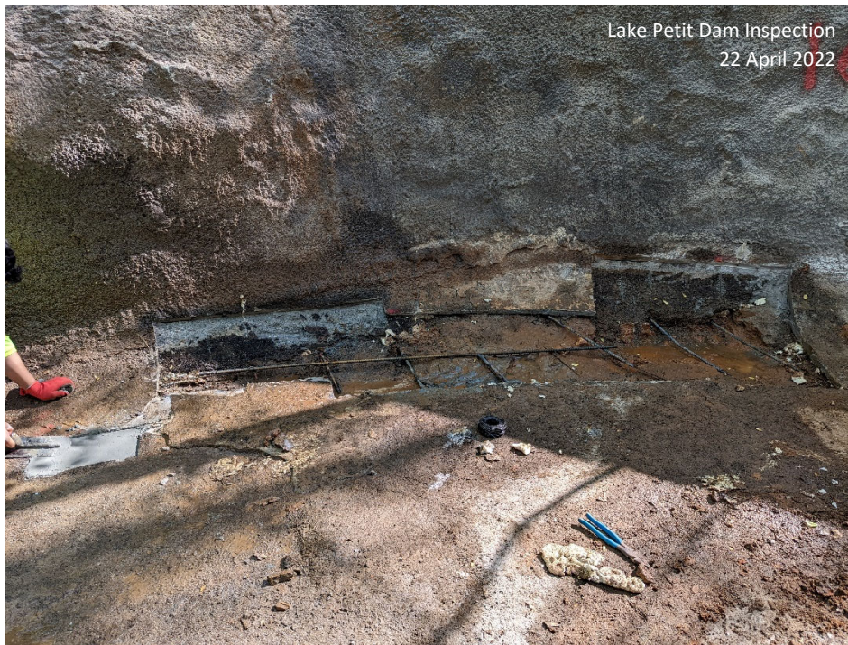
Photograph 37: Repair at Step 16 – rebar installation
