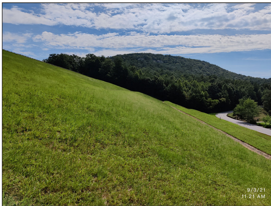
Photograph 2: Downstream Face, Sept. 2021 – overview of downstream face in good condition
