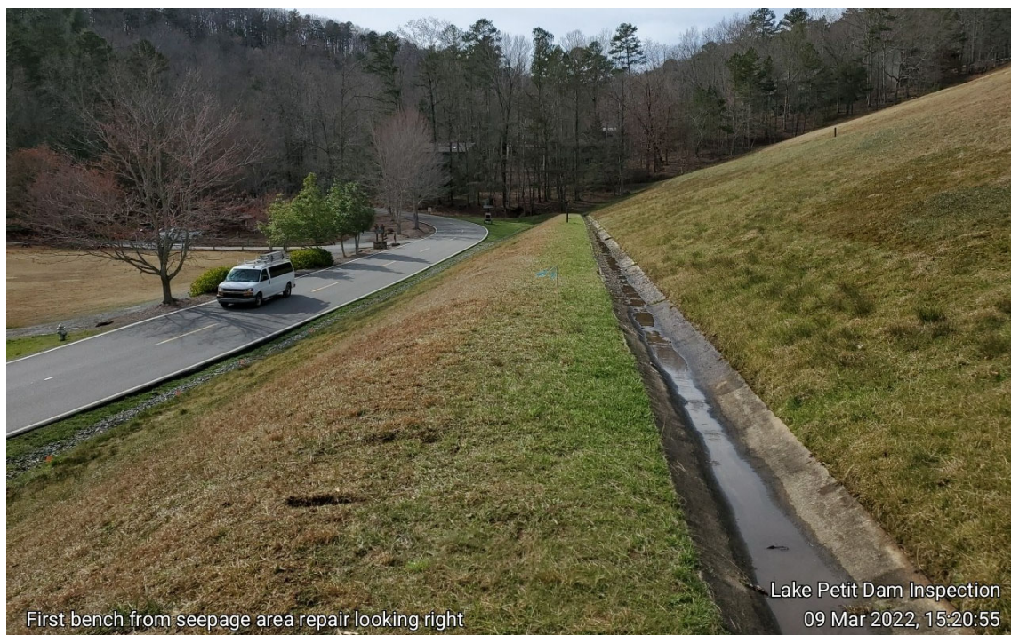
Photograph 12: Bench 1 (El. 1544) looking toward right abutment
