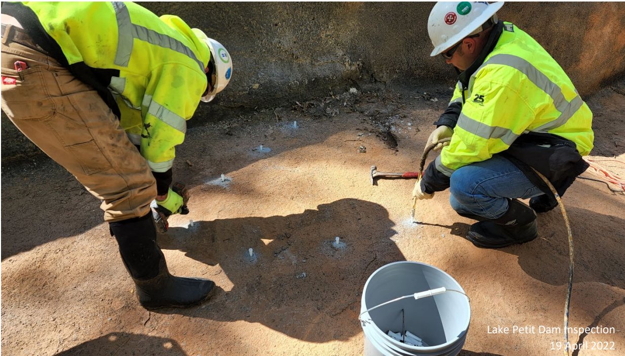
Photograph 33: Hydrophobic polyurethane grout injection into void under spillway chute
