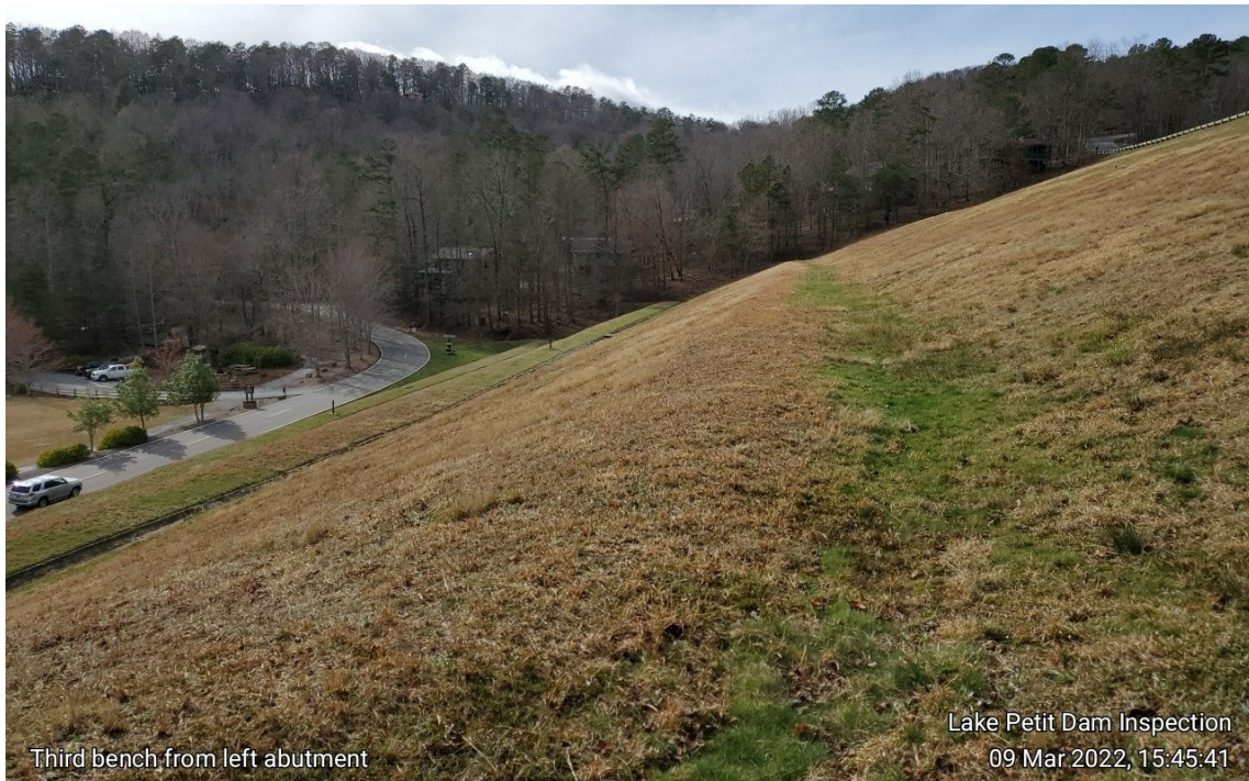
Photograph 19: Bench 3 (El. 1584) looking toward right abutment
