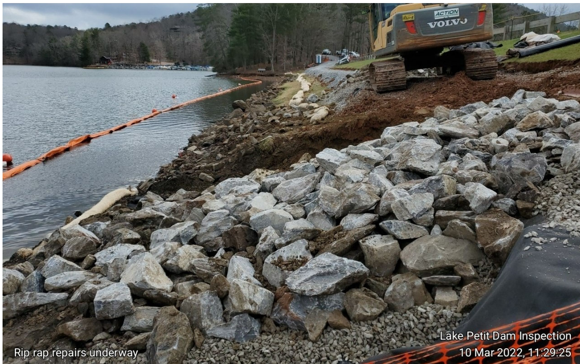
Photograph 1: Beginning of shoreline protection repairs (looking toward left abutment)
