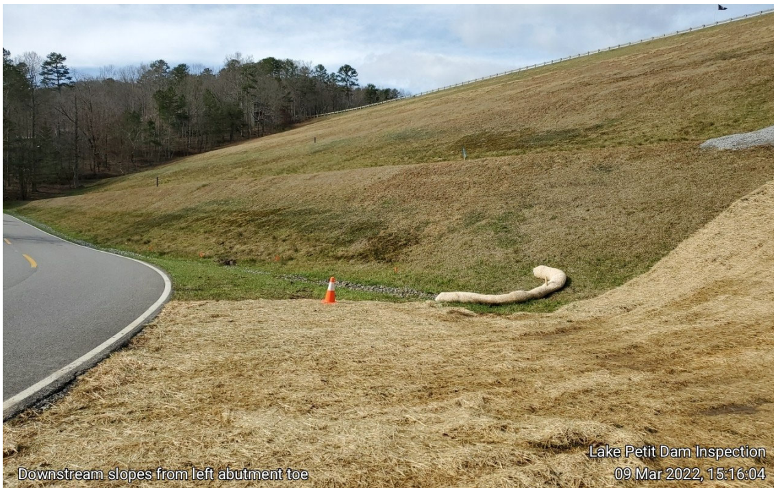
Photograph 11: Downstream toe from left abutment
