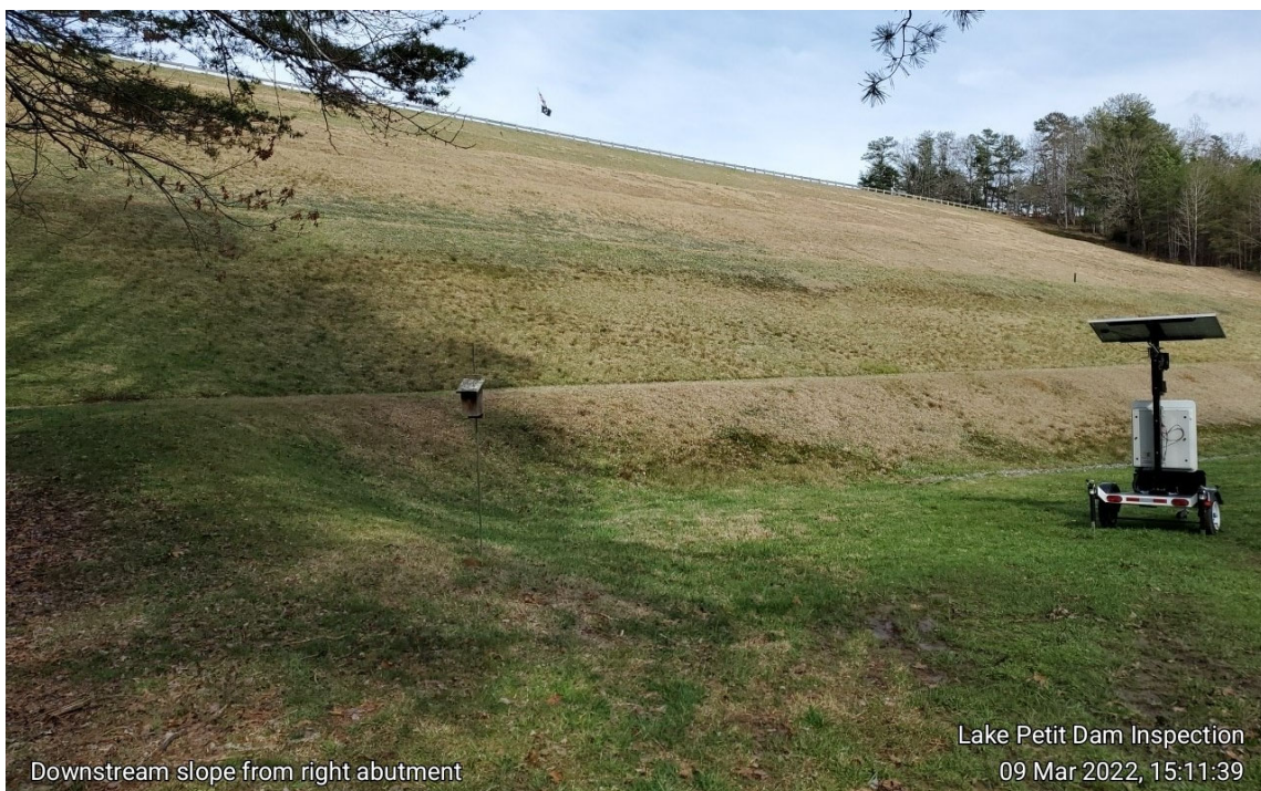
Photograph 10: Downstream slope from right abutment
