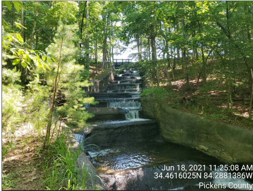
Photograph 3: Spillway, Jun. 2021 – general view of stepped spillway with moderate flow. Downed trees previously identified across or within the spillway were observed to have been removed.
