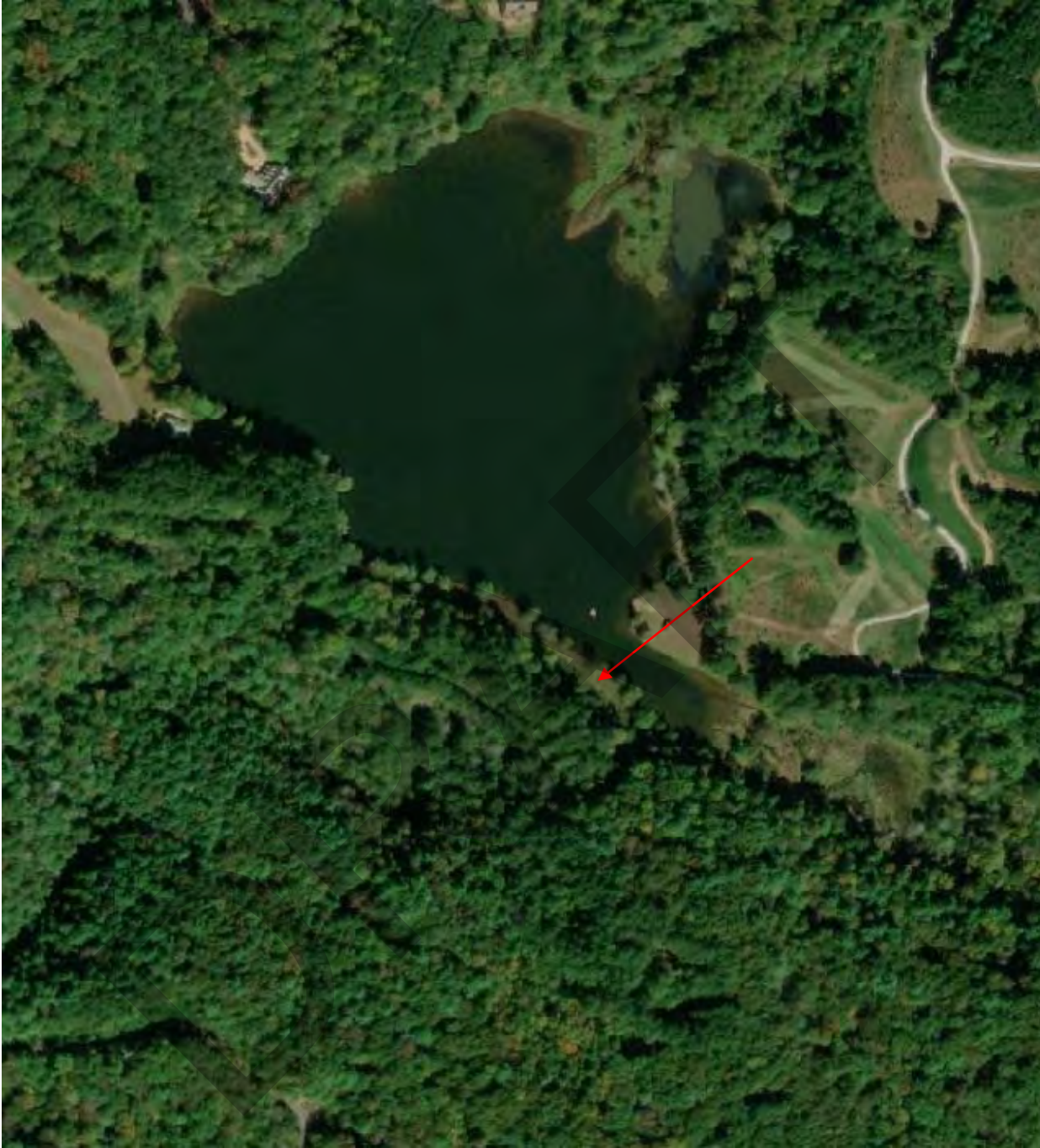
Lake Cox Dam
