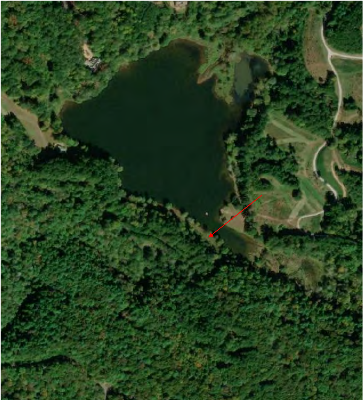
Lake Cox Dam
