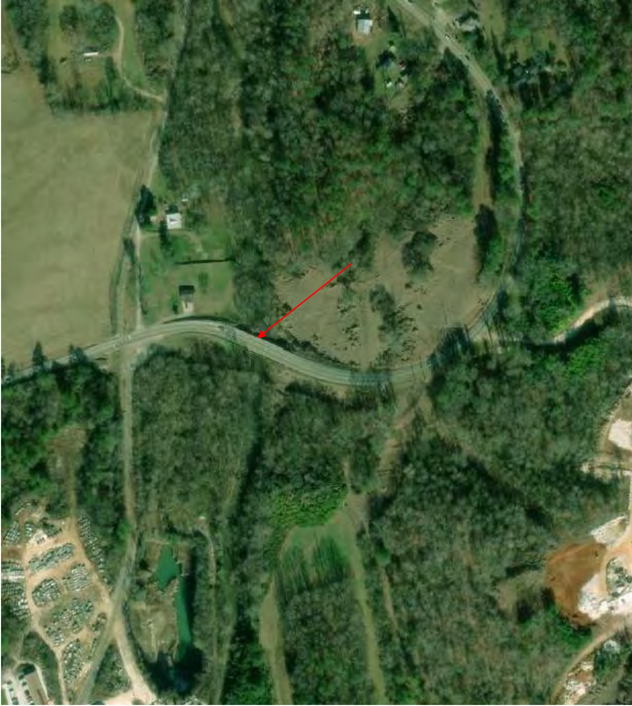
State Route 53 (Near Marbleblock Lane)
