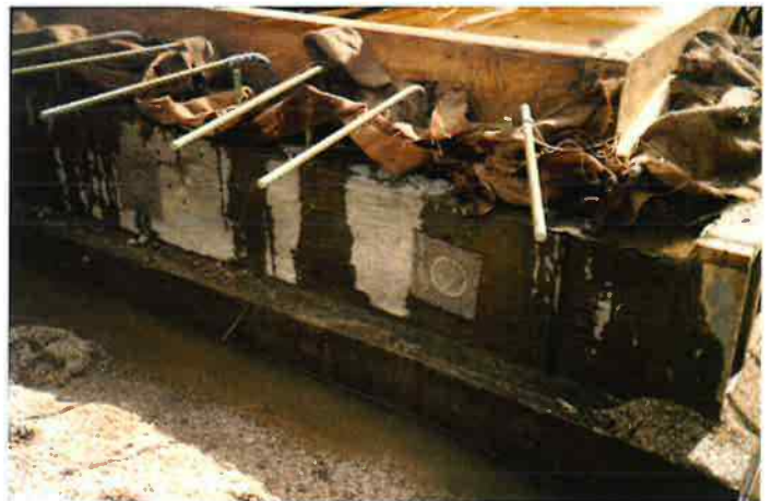
Weep holes with screens to control seepage.
