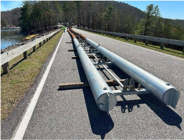
Floats and stem laid on road prior to installation.
