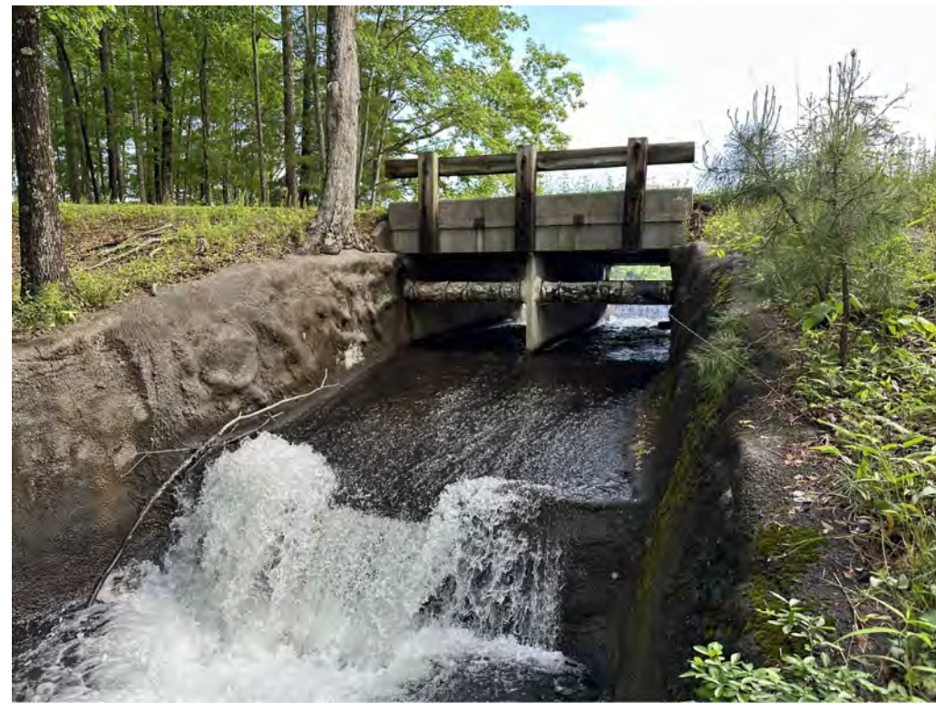
1 EXISTING CONDITIONS 6 TOP CREST OF SPILLWAY
