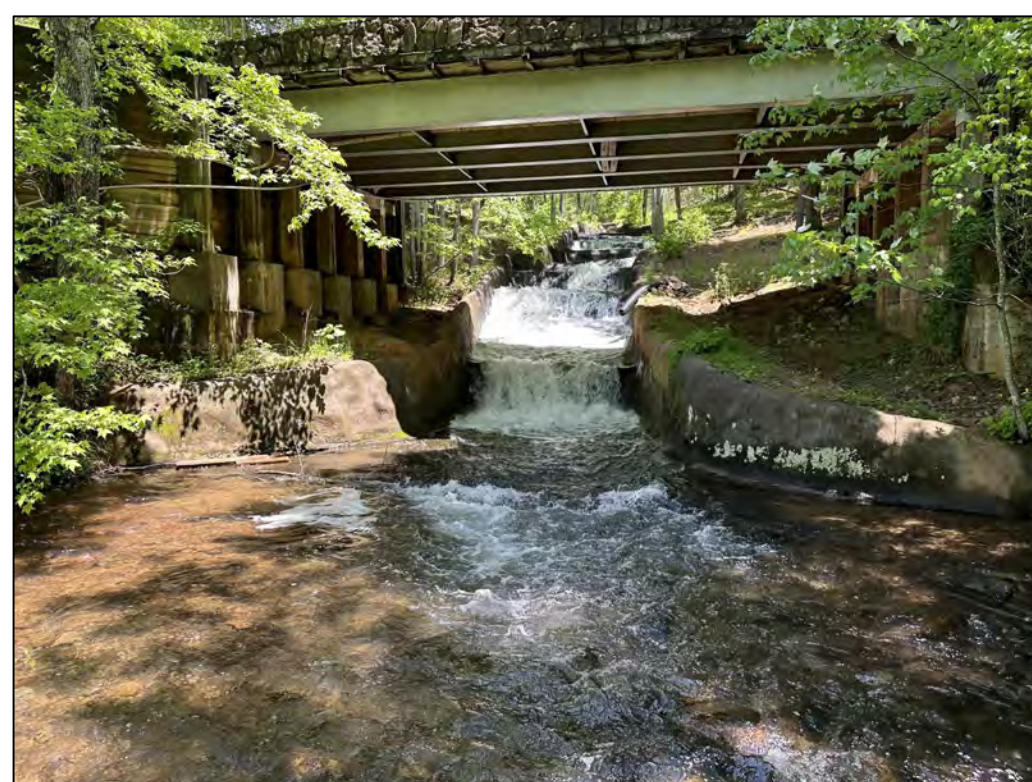
3 EXISTING CONDITIONS 6 BOTTOM OF SPILLWAY
